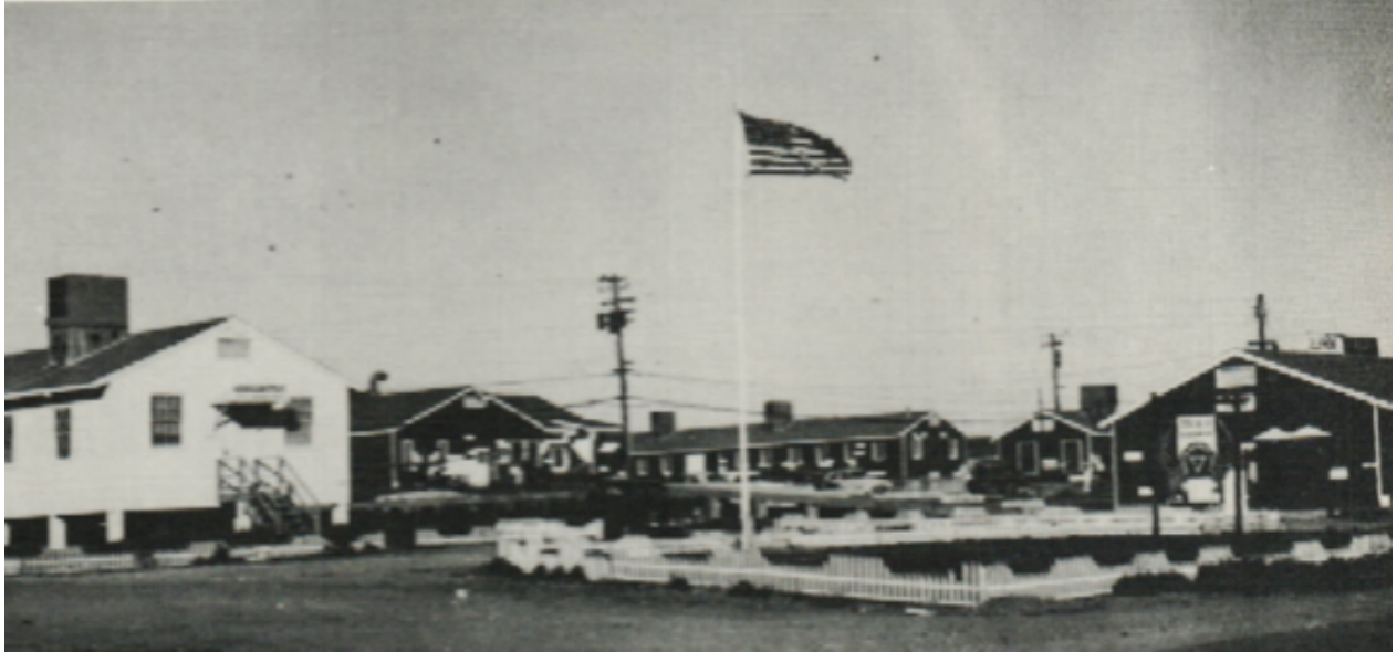
2275 ABG compound, Beale AFB, CA
